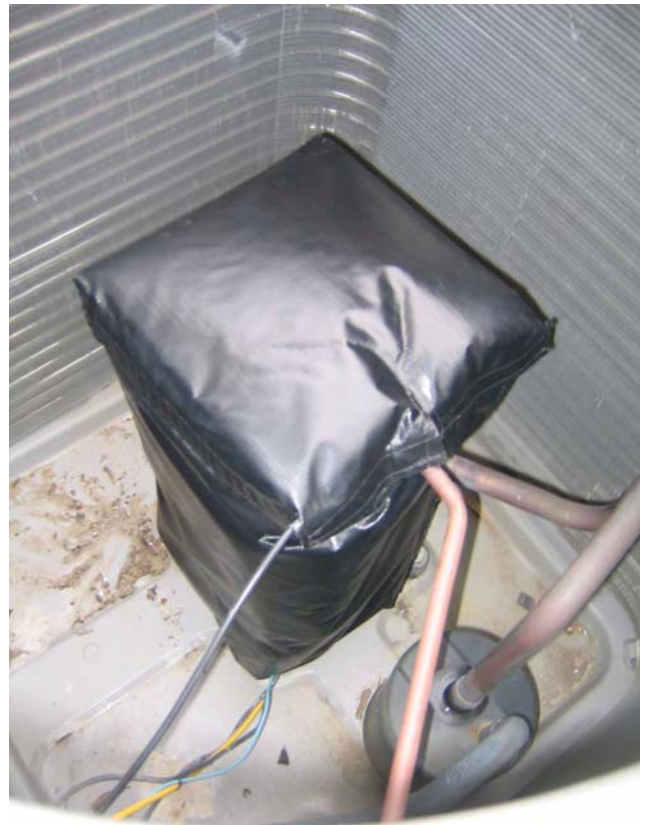
Photo captions clockwise from upper left: 1) Blanket flat layout before folding in to shape 2) Assembled blanket 3) Taking measurements with SPL meter 4) Blanket installed over compressor
