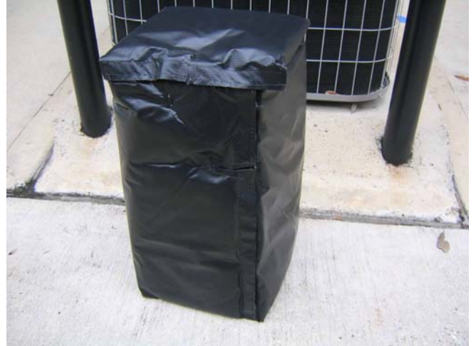
Photo captions clockwise from upper left: 1) Blanket flat layout before folding in to shape 2) Assembled blanket 3) Taking measurements with SPL meter 4) Blanket installed over compressor
